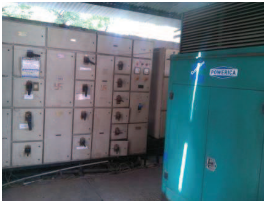
Photo : Power Supply Unit with Generator
