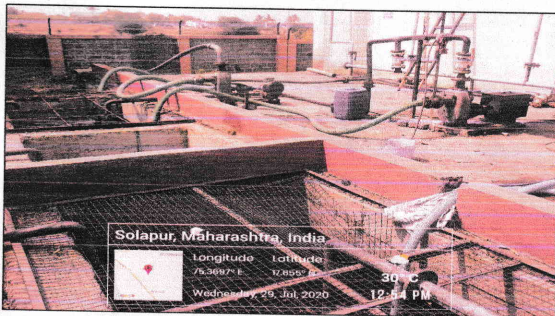
Existing STP plant
