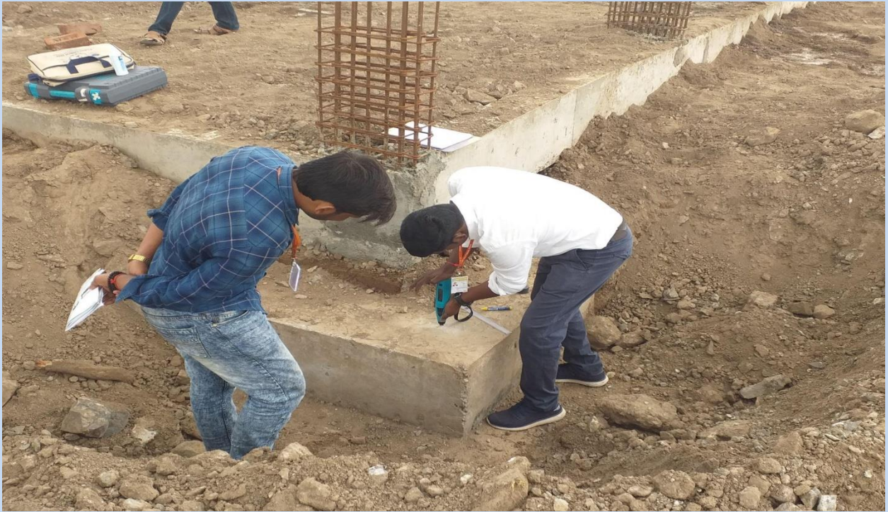
Finding Compressive Strength by Rebound Hammer through Non Destructive Testing
