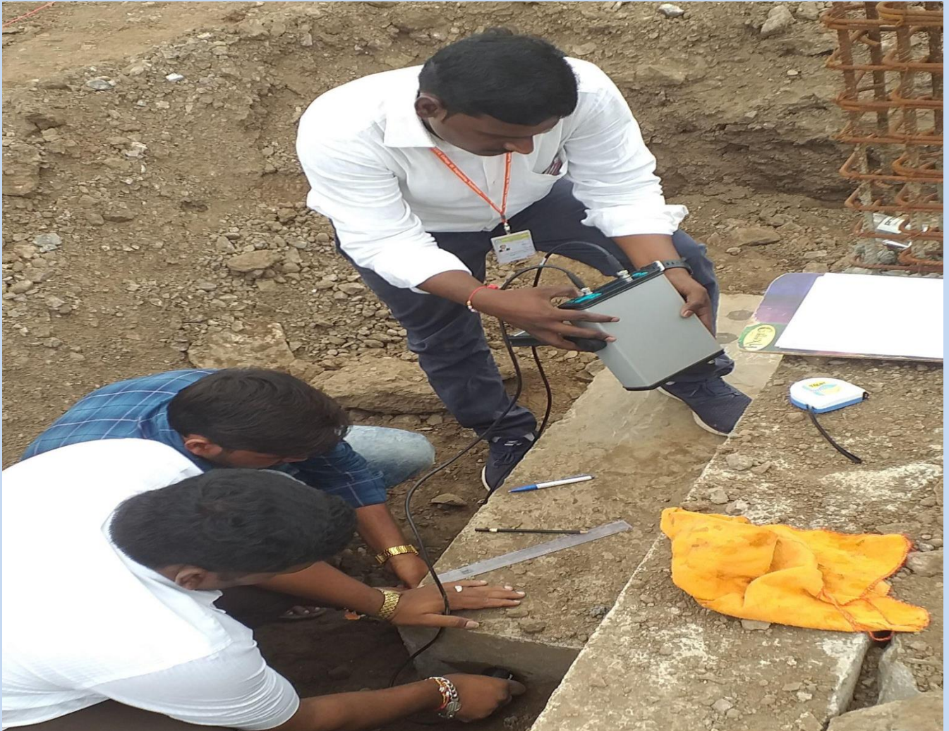
Finding quality of Concrete by ultrasonic pulse velocity meter
