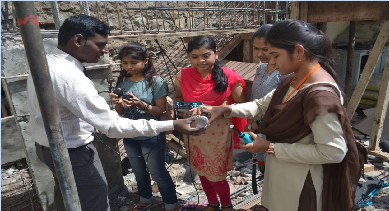
Finding quality of Concrete by ultrasonic pulse velocity meter
