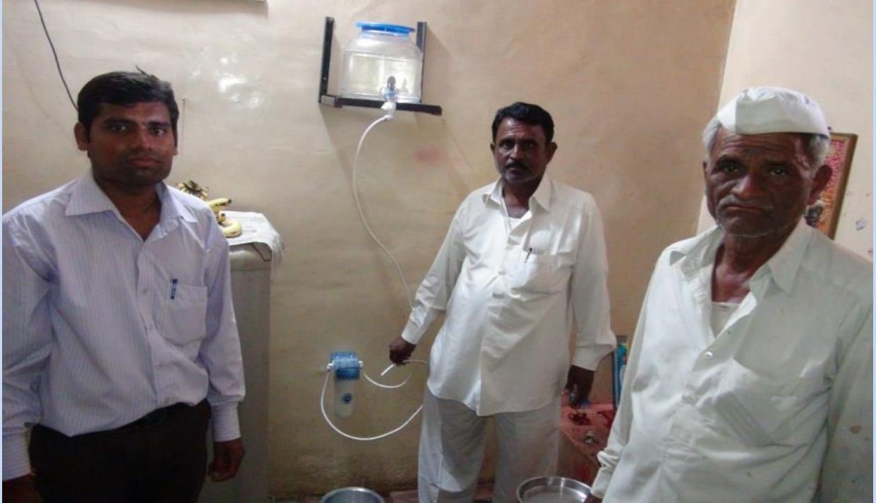
Installation of Water Filter
