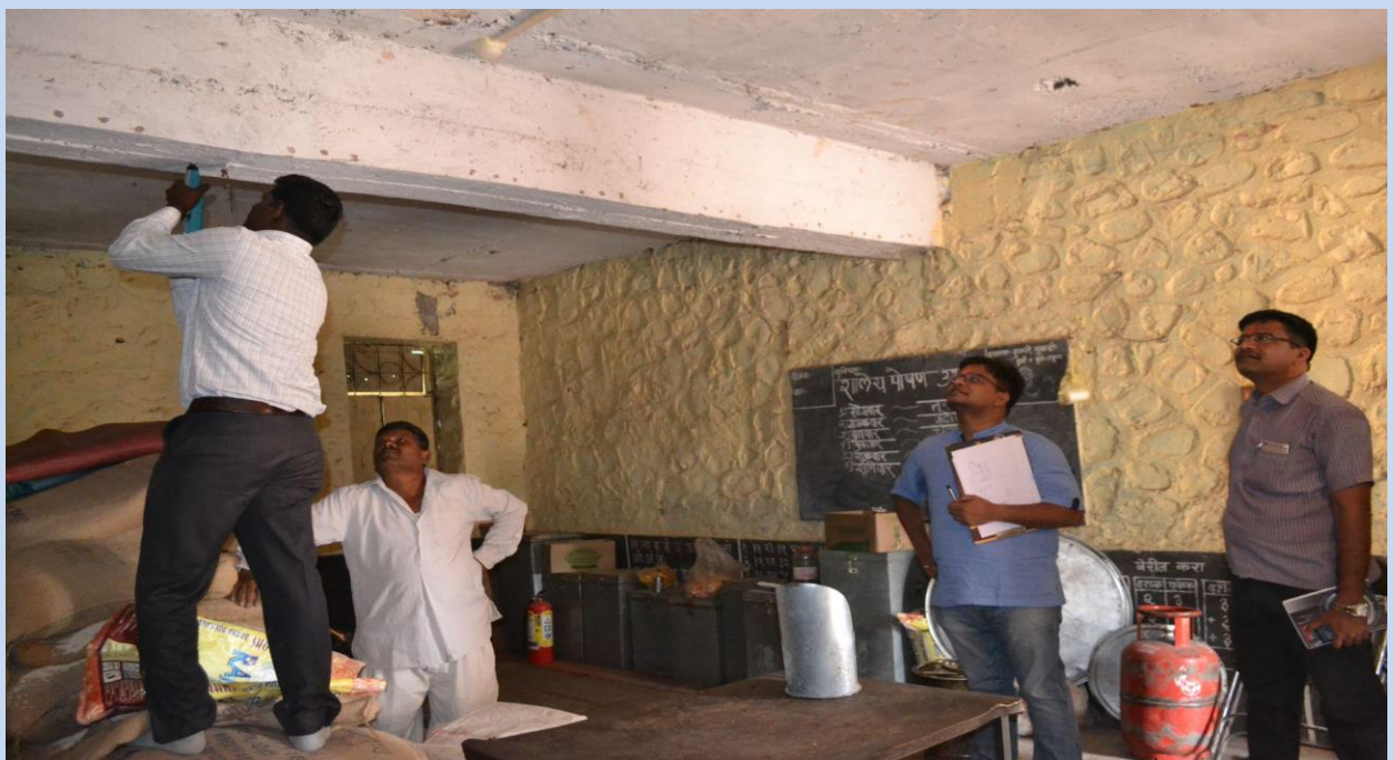
Structural Audit of Zilha Parishad primary School
